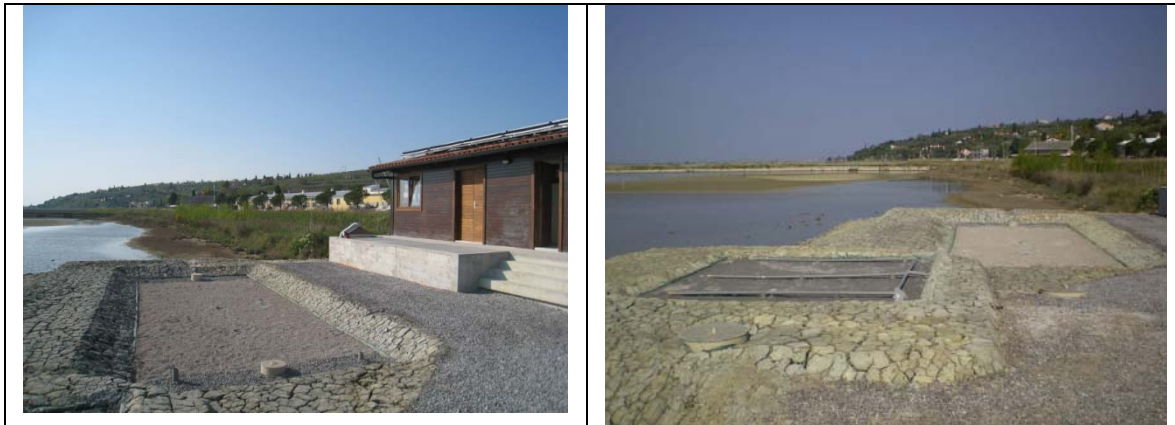
Figure 1 Soline Sanbox prototype with constructed wetland for graywater treatment.
