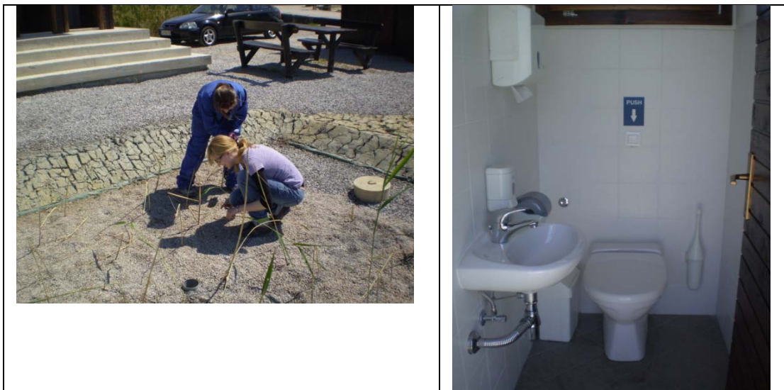
Figure 2 Planting of constructed wetland in March 2011, vacuum toilets.
